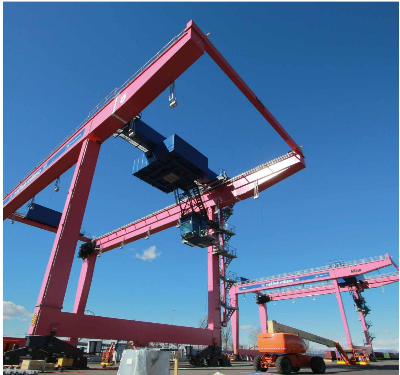
Erection of the new RMGs (Railway Mounted Gantry Cranes) at Rail Hub Milano in Melzo, northern Italy.
